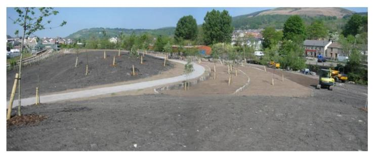
To reinforce the sites links with the past, more than a thousand reclaimed concrete railway sleepers have been set vertically to create retaining structures for planted and seeded terraces.
