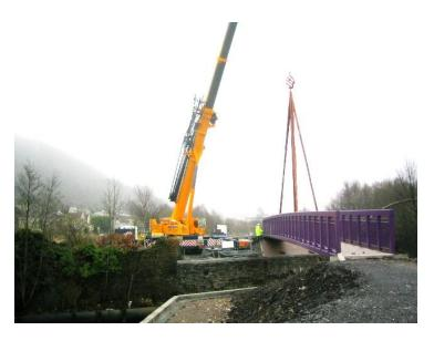
Phase two involved building two large in-situ concrete bridge abutments faced with Pennant Sandstone and installing a 31 metre span cycle and footbridge over the river Cynon. A temporary road was constructed to provide access for the 200 tonne crane.
