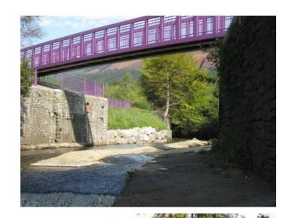
Before we could install the bridge we were required to break out the central stone pier of a former bridge which required us to undertake quite major work within the river where access was extremely difficult.
